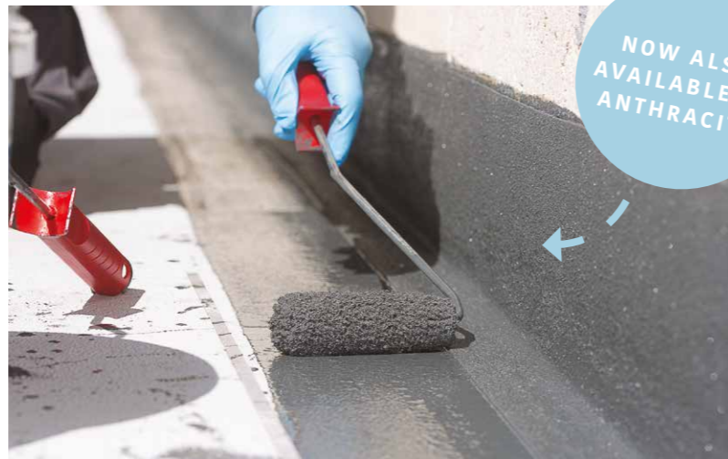
The liquid waterproofing is suitable for connections, structural details and surfaces, in both new construction and renovation.
