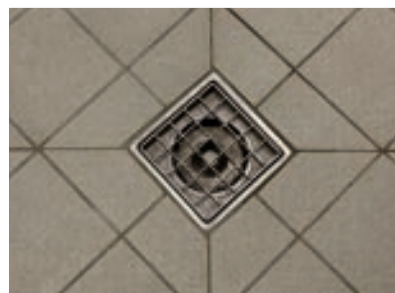
All gutters were seamlessly incorporated into the waterproof membrane.
