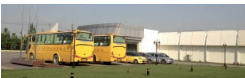
6,000 m 2 roof at Nanjing MeiRui Pharma was waterproofed using KEMPEROL® V 210.
