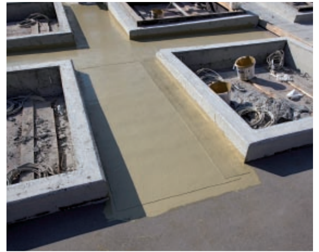
During application: all skylights and the surfaces between them were carefully waterproofed and sealed with KEMPEROL® 2K-PUR.
