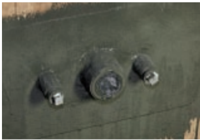
Because the waterproofing is applied as a liquid, all joints, pipes and drains can be seamlessly incorporated in the homogenous membrane.
