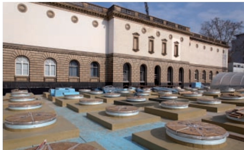
The insulation was laid on top of the waterproofing system.
