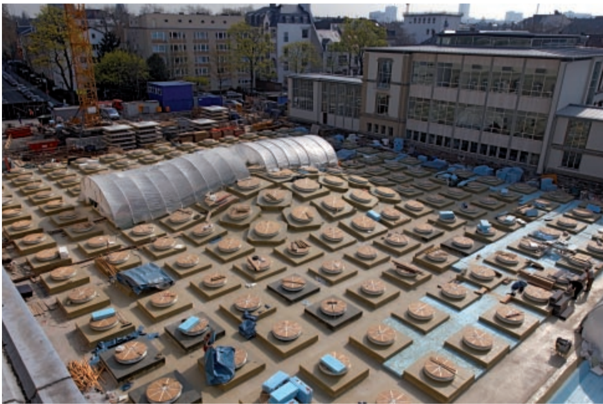
The architects' product of choice for waterproofing the roof area and the 195 skylights was KEMPEROL®.
