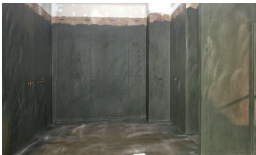
Both floors and walls were waterproofed with KEMPEROL®.
