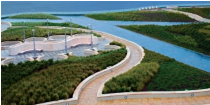
The 114 ft. elevation which includes the Sky Garden is a tapestry of surfaces protected by KEMPER SYSTEM waterproofing from below: Landscaped areas, decorative concrete, pedestal pavers, flagstone, and pebble tile. The liquid-applied membrane was ideal for sealing around penetrations.
