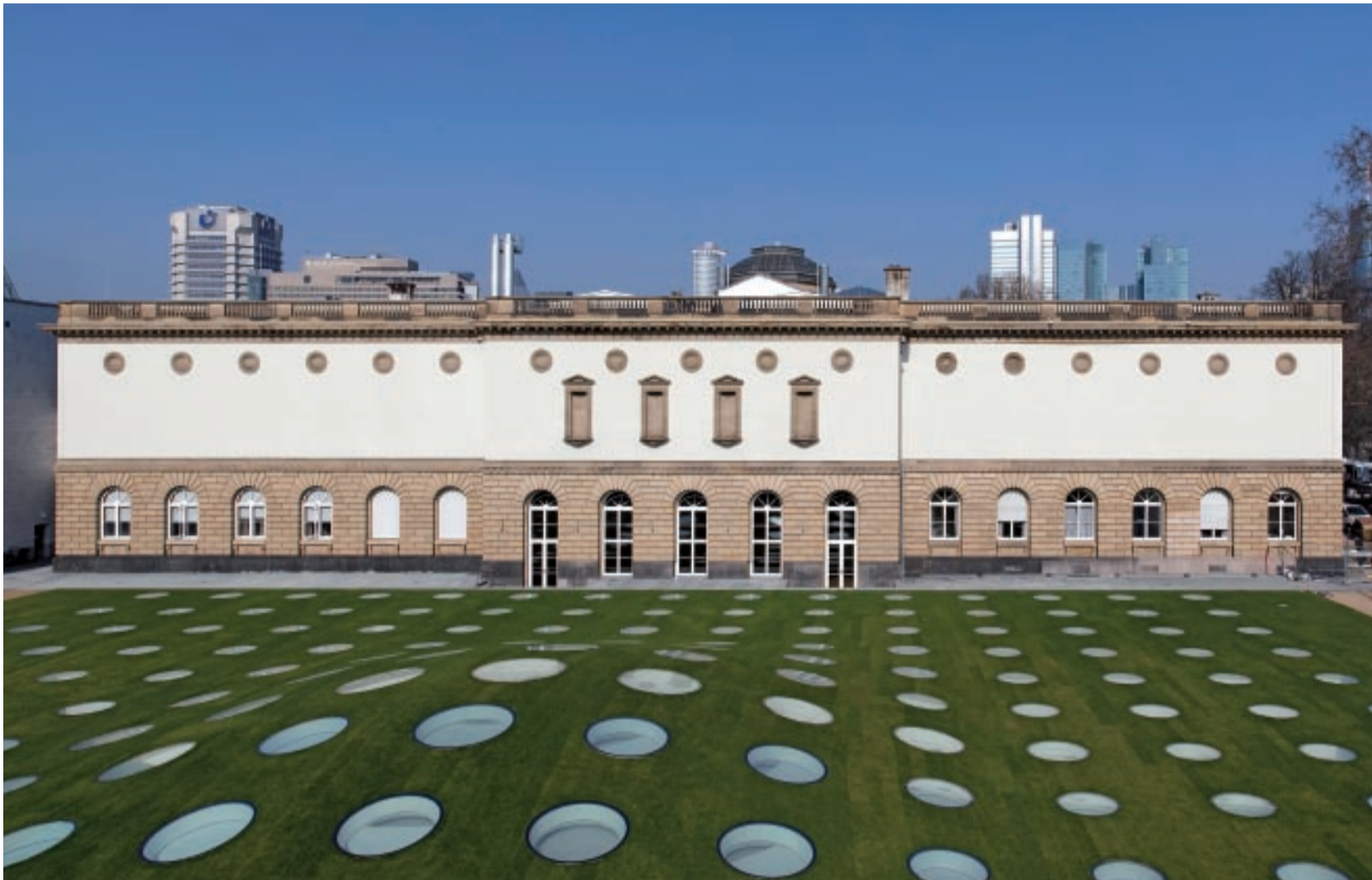
The skylights indicate the exhibition space: the new extension of the Städel Museum is underground beneath the garden area.
