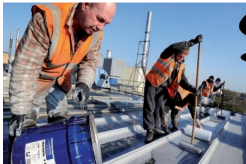
Applying KEMPEROL® V 210 to the metal standing seam roof
