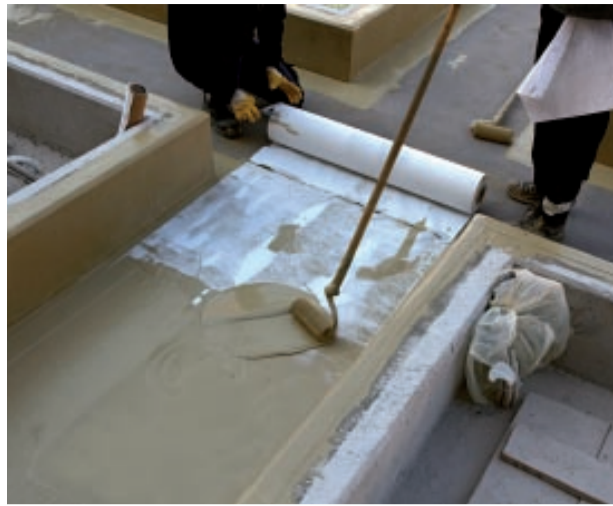
During application: all skylights and the surfaces between them were carefully waterproofed and sealed with KEMPEROL® 2K-PUR.
