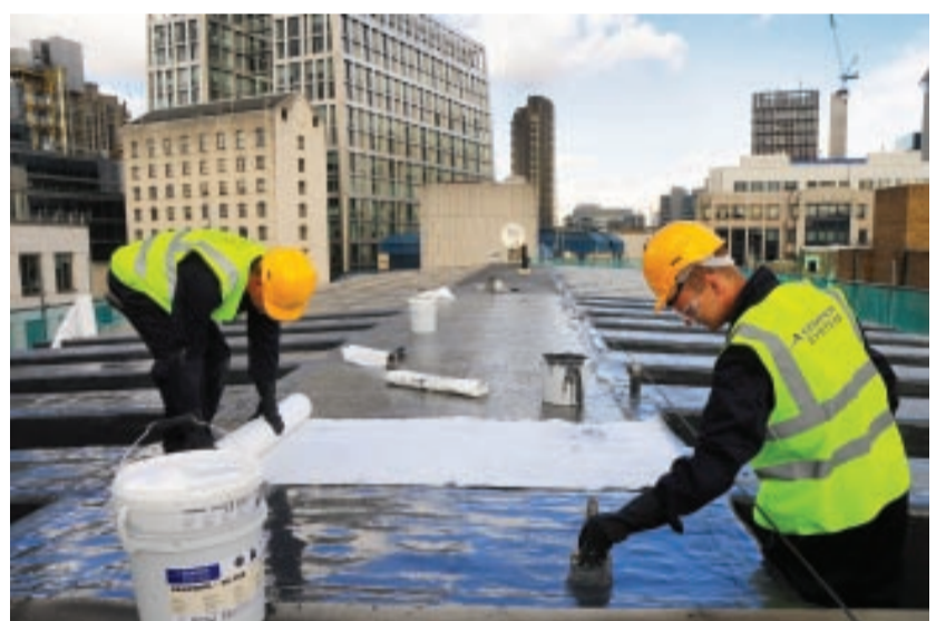
The complex roof of the Guildhall
