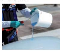
The ready-for-use KEMPEROL® FALLSTOP coating is then applied evenly and free of bubbles in four steps using a foam roller in a criss-cross fashion.
