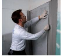
3 Reinforcement fleece covers all small cracks..
