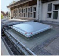
The first skylight dome coated with KEM-PEROL<sup>®</sup> FALLSTOP was installed as a sample for final approval and waterproofed with KEMPEROL<sup>®</sup> 2K-PUR
