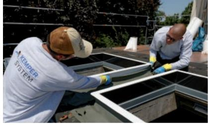
question arose as to how fall-through Waterproofing takes place in a confined space. The reinforcement fleece soaked in KEMPEROL® is applied directly to the sanded bitumen sheeting.
